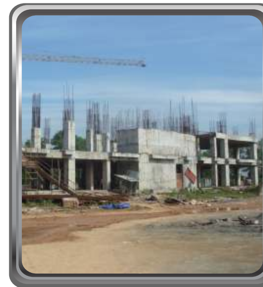
IT Building working progress Ready to Occupy by 2015
