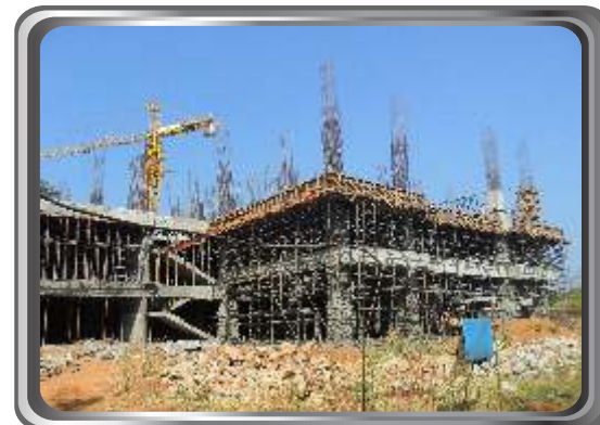
Construction of Multi-storeyed IT Block at Infopark Thrissur in Progress.
